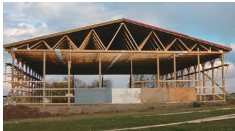
Photo 6.3 Because roof trusses, such as those shown, require support only at their ends, it is possible to construct buildings with large, unobstructed floor areas.
